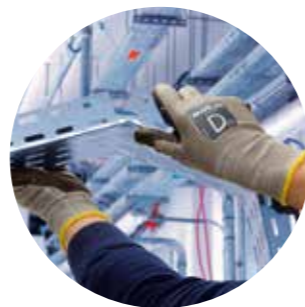
Cable path handling
